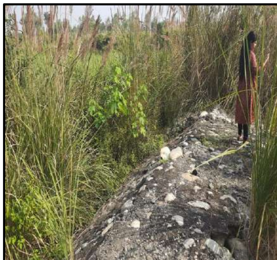
Figure 4 Bunds at Pur ka Tanda
