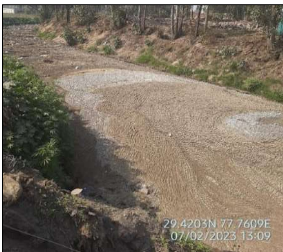
Figure 53 Sludge blanket formation observed in Dhandera drain at Jansath Road, Muzaffarnagar
