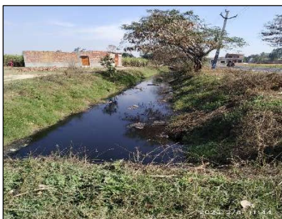
Figure 60 Mansoorpur drain near Husenpur Bopara village
