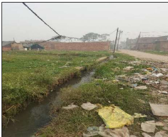
Figure 37 Drain carrying sewage of Suzroo village
