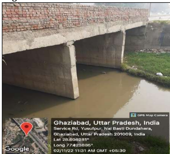
Figure 96 Gaur city drain
