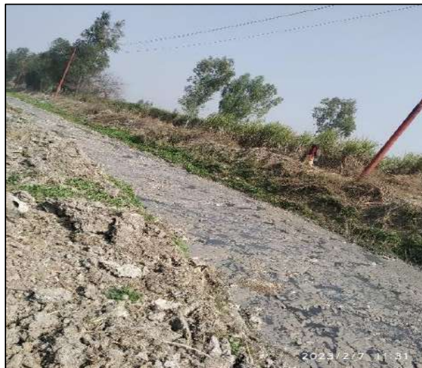
Figure 47 Sludge deposition in Jat Mujheda drain
