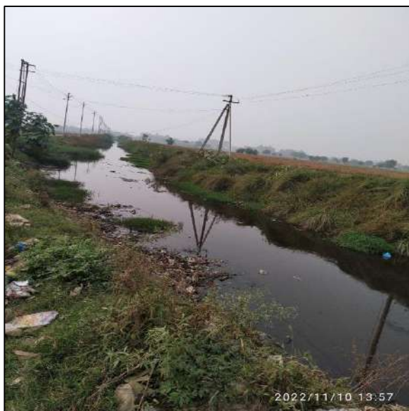
Figure 88 Bhoorgarhi – Kalugarhi confluence drain
